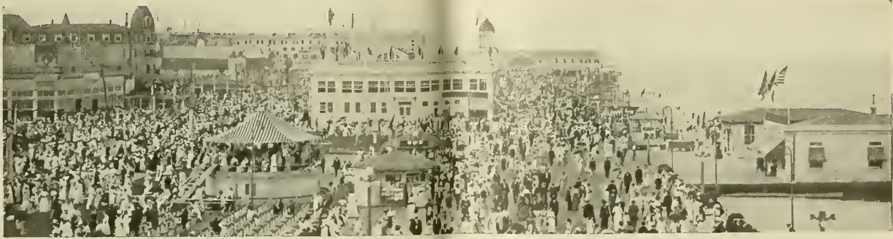
ASBURY PARK BOARDWALK
